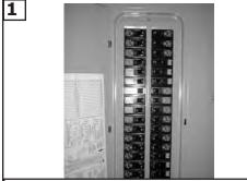
Before you begin installing the fan, Switch power off at Service panel and lock service disconnecting means to prevent power from being switched on accidentally. When the service disconnecting means cannot be locked, securely fasten a prominent warning device, such as a tag, to the service panel.
